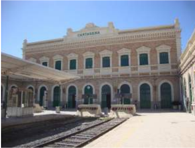
Fachada principal andenes
